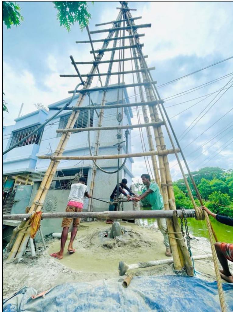
Figure 3. Deep Tubewell Installation Process
