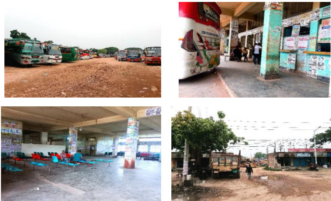
Figure 2: Existing Conditions of Nawdapara Bus Terminal
