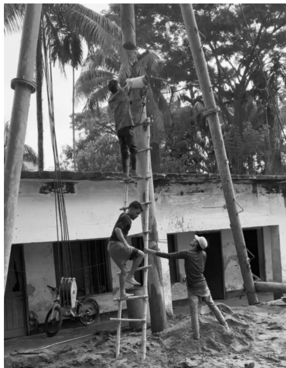
Figure 5: Sand Compaction Pile Work
