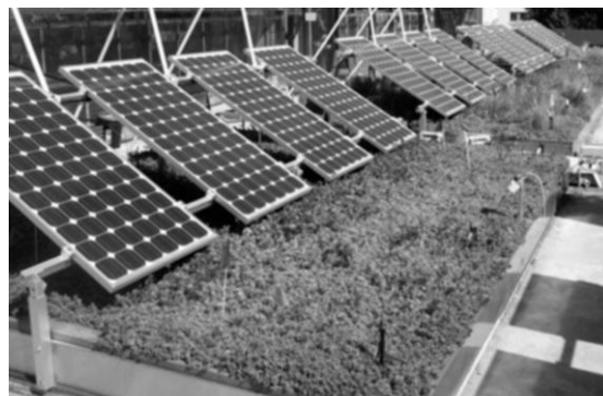
Figure 4. Green roof mounted with rooftop solar photovoltaic(PV) systems. Source: ( Zheng and Weng, 2020 )
