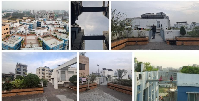
Figure 10: Overview of the Interconnected Rooftops in Assurance City (Source: Field Survey, 2024)
