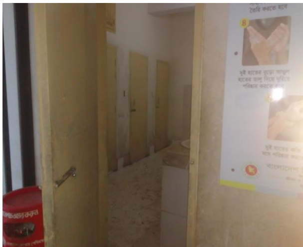
Figure 3: Existing 2nd class toilet an Wash area at Khulna railway station
