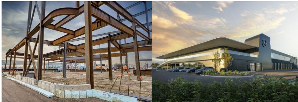
(a) Construction Stage
