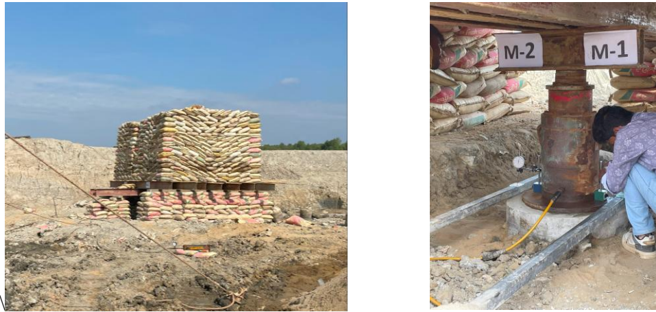
Figure 1: Pictures of pile load test (ASTM D-1143-07).
