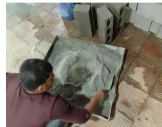
(c) mixing of mortar
