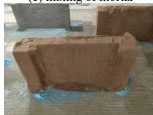
(f) curing of brickwall
