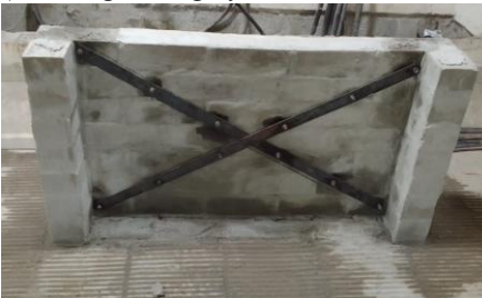
(c) Strengthening by Mild Steel Plate
